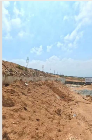
Photo 15 · 0:52 into the visit retaining wall
