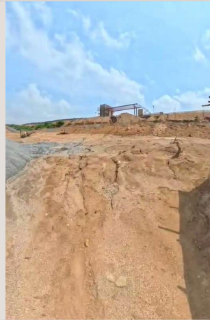
Photo 10 · 0:34 into the visit No note recorded
