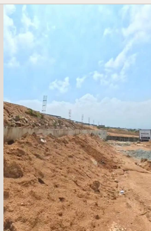
Photo 15 · 0:52 into the visit retaining wall
